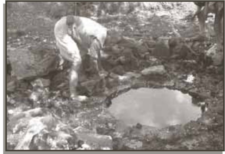
Making an intake tank without cement, Jajarkot, Nepal
