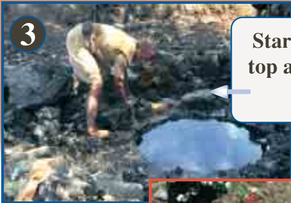
Leaving a hole big enough for a person to fit in, the lid is made.
