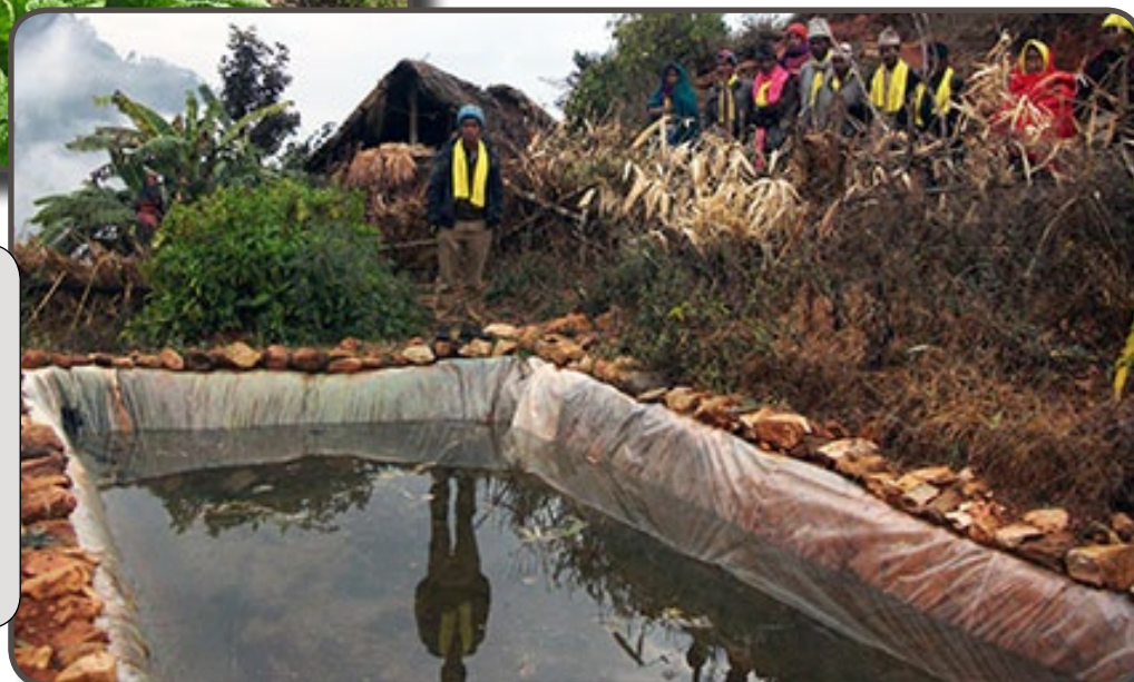
Right - the Humlis view a polythene-lined irrigation pond built last year in Bhalim village, where water is collected from a small spring for irrigating paddy fields, fruit trees, kitchen gardens and home nurseries.
