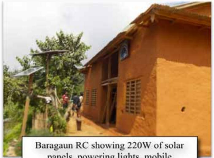
Baragaun RC showing 220W of solar panels, powering lights, mobile charging, laptops and digital projector
