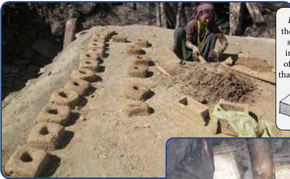
Left - preparing bricks for making the chimney component of smokeless stoves. The bricks are made by filling a form with mud. In the middle of the form is a round piece of wood that leaves the hole. The bricks, after 48
